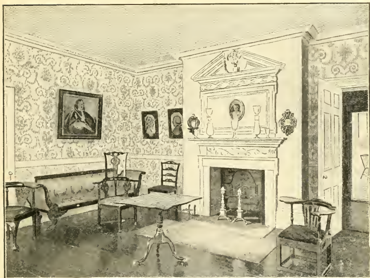
Colonial parlor (restoration).
